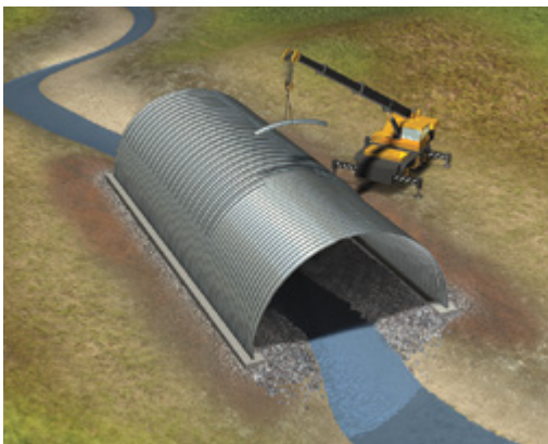
If specified, reinforcement ribs are then added.
